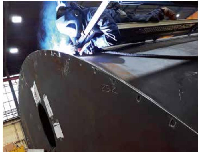
Segmentdeur under construction.
