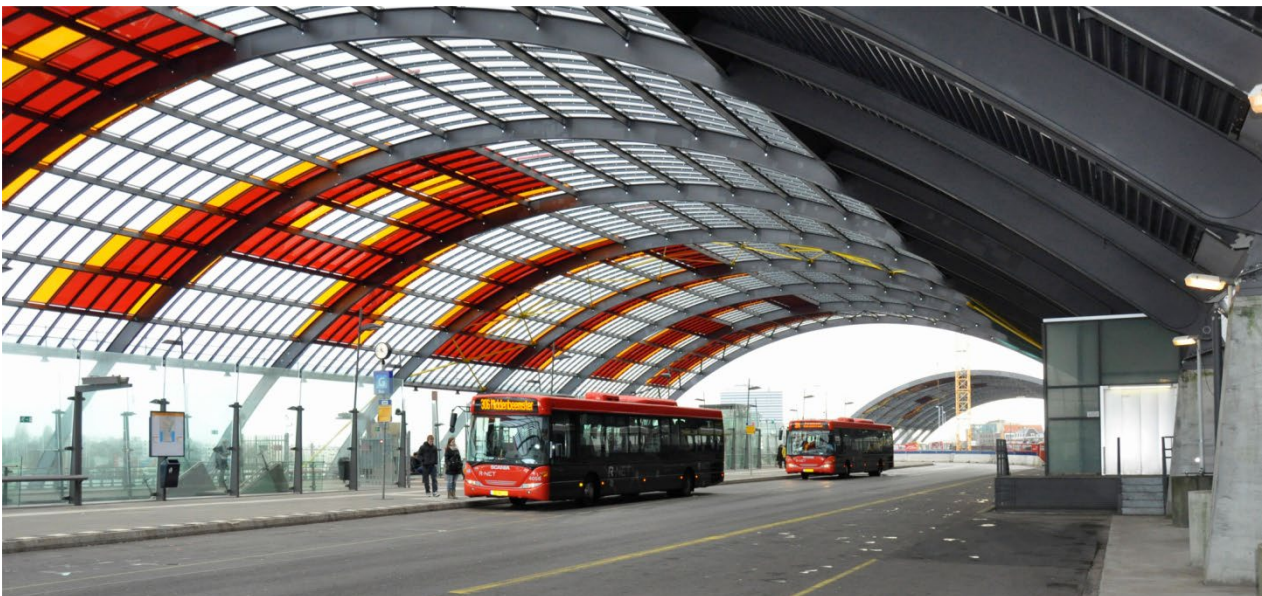
Fig. 9 Coloured plastic film inserted into some of the cold-bent glass panels will form the word AMSTERDAM once the canopy is complete.
