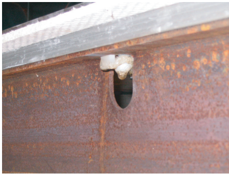
Fig. 9: The nylon bolt softens
