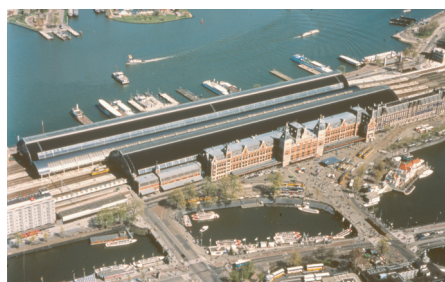
Fig. 1: Aerial photo of Amsterdam Central station as it is without the bus station roof (Photographer: Dick Sellenraad)
